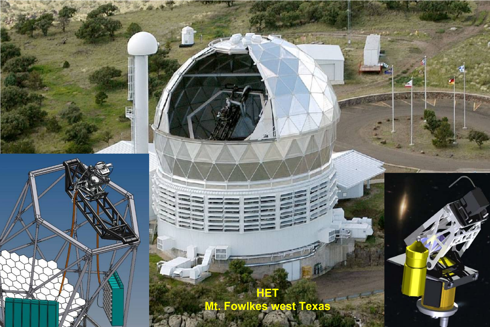
VIRUS consists of 150 units mounted on HET
